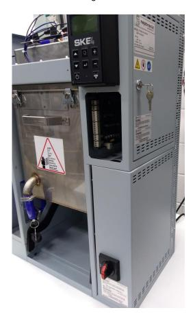
**1.3.** Open the access door to the low voltage compartment, located on the top right side of the cabinet, by using the humidifier access key.
